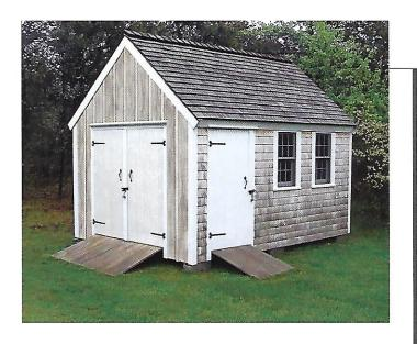
The rustic, natural beauty of red cedar is display in this attractive 10-ft. by 14-ft. workshow Cedar shingles cover the sidewalls; the roof made of cedar shakes. The gable wall is sided with cedar board-and-batten siding.
