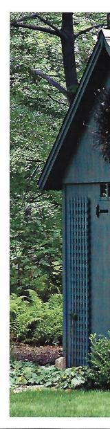
This charming backyard building features cedar clapboards on the sidewall, board-andbatten siding on the gable end wall, and asphalt shingles on the roof. It measures 12 ft. by 14 ft., which is an ideal size for use as a storage building, garden shed, or kid's playhouse.
