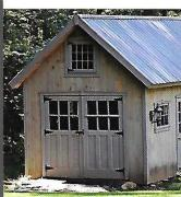
A Built as a tractor barn this 12-ft. by 22-ft. outbuilding features vertical-board siding, standing-seam metal roof, and doublewide doors salvaged from an old dairy barn. The upper window on the gable end wall provid access to an overhead storage loft.
